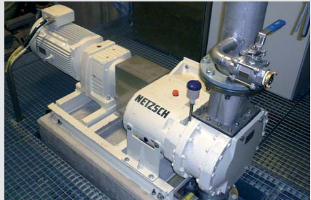
A TORNADO® pump in a paper factory for unloading Kaolin from tankers. Flow rate is 330 gpm (75 m 3 /h) and pressure is 60 psi (4 bar).
