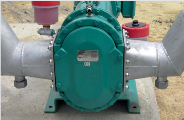
Feed pump for a biogas substrate. Flow rate up to 175 gpm (40 m 3 /h) at a pressure of 30 psi (2 bar).
