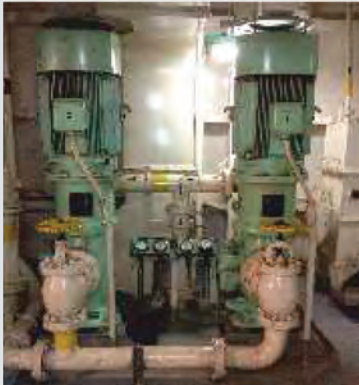
Lubricant oil, 660 gpm / 150 m 3 /h 60 psi / 4 bar Pump installed inside the vessel
