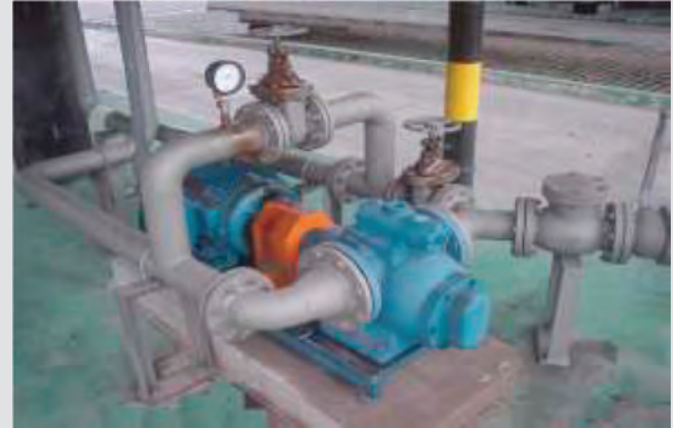
Lubricant oil 260 gpm / 60 m 3 /h 120 psi / 8 bar
